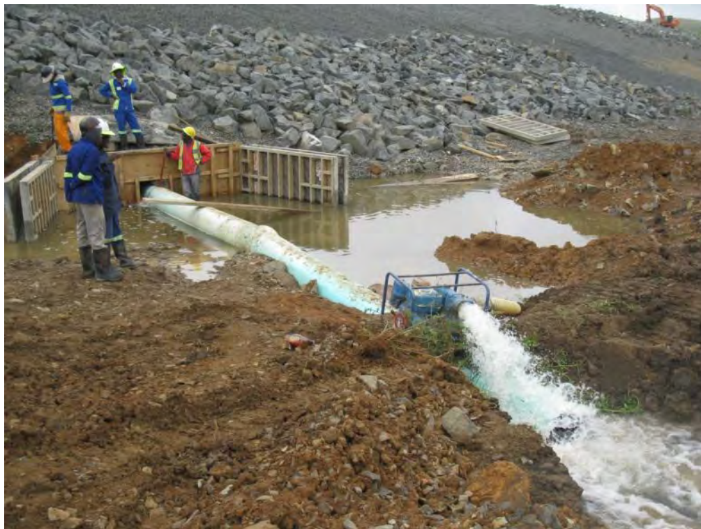
Figure 16: Dewatering directly into watercourse
