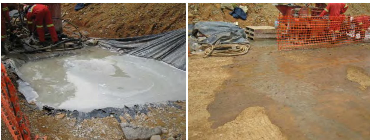
Figure 20: Improper wastewater management
