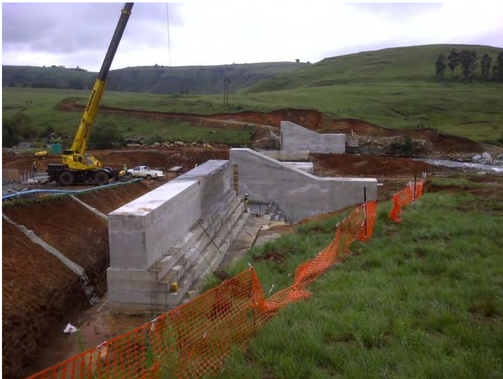
Figure 5: Construction of the fish barrier
