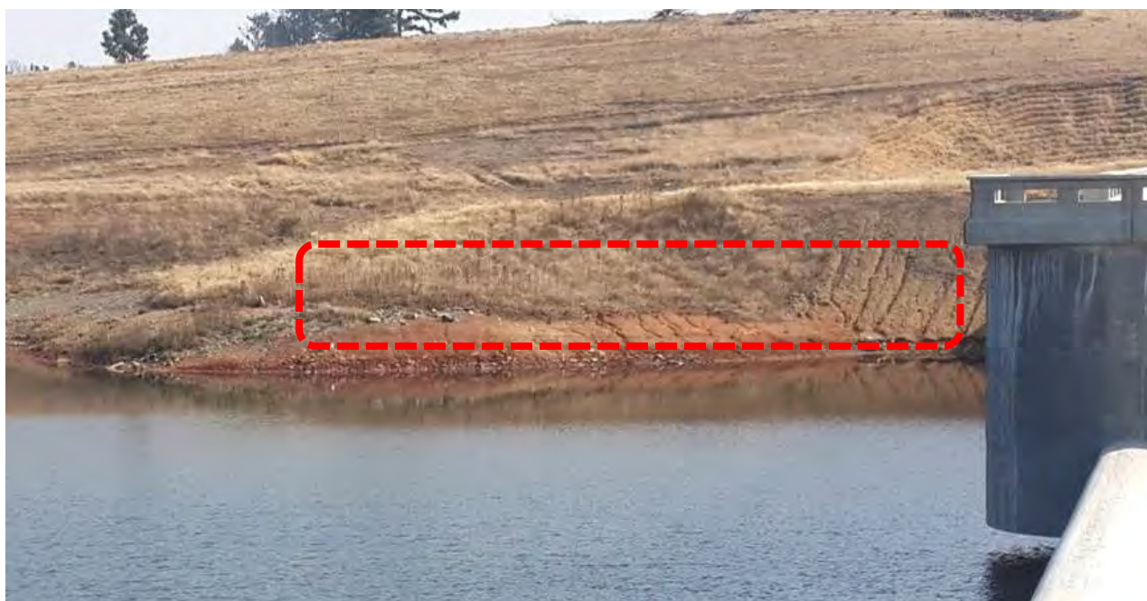
Figure 10: Bare area - upstream left bank at dam wall
