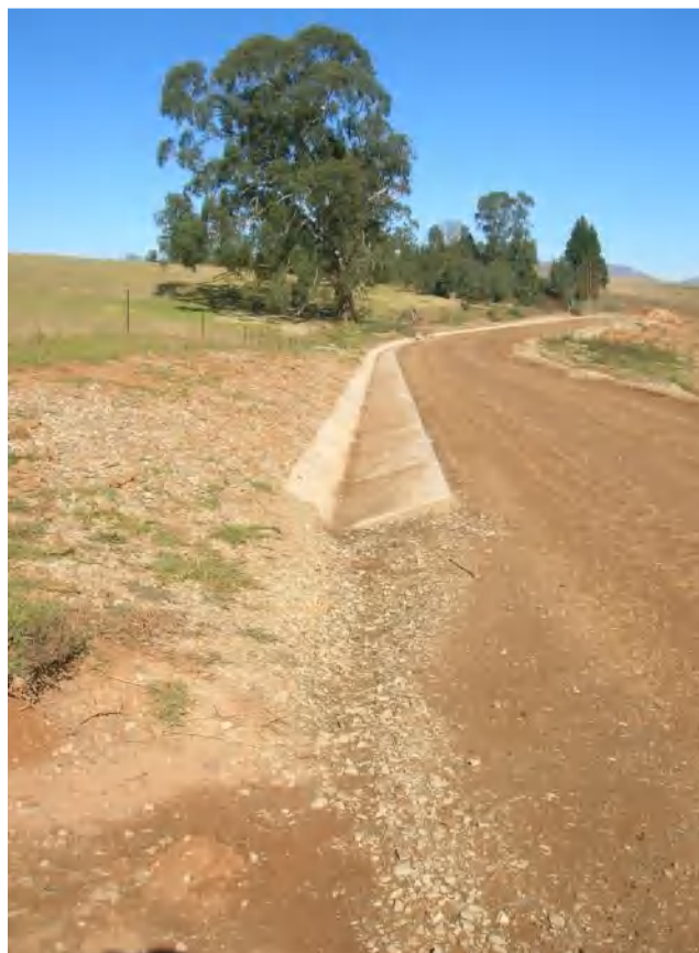
Figure 3: Concrete drainage channel
