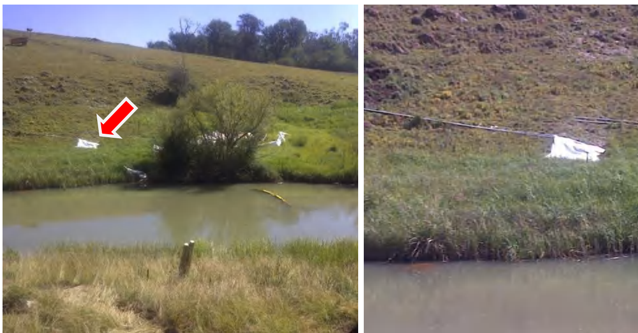
Figure 11: Dewatering through silt socks
