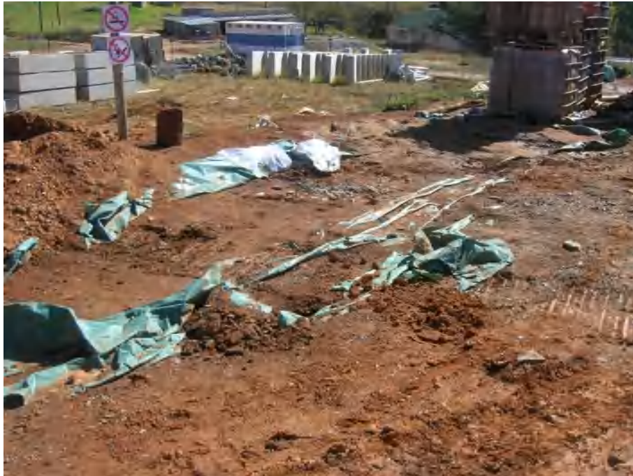
Figure 18: Repair bunded area used to contain diesel bowers
