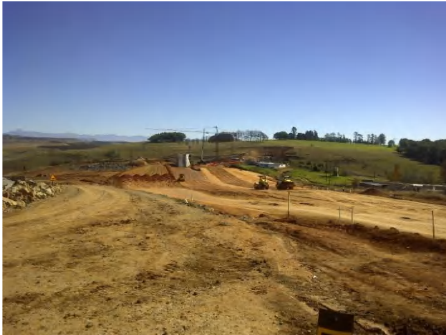
Figure 2: Backfilling of earth embankment
