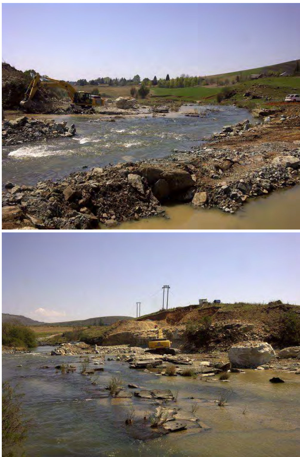
Figure 20: No provision for management of siltation at fish barrier instream works
