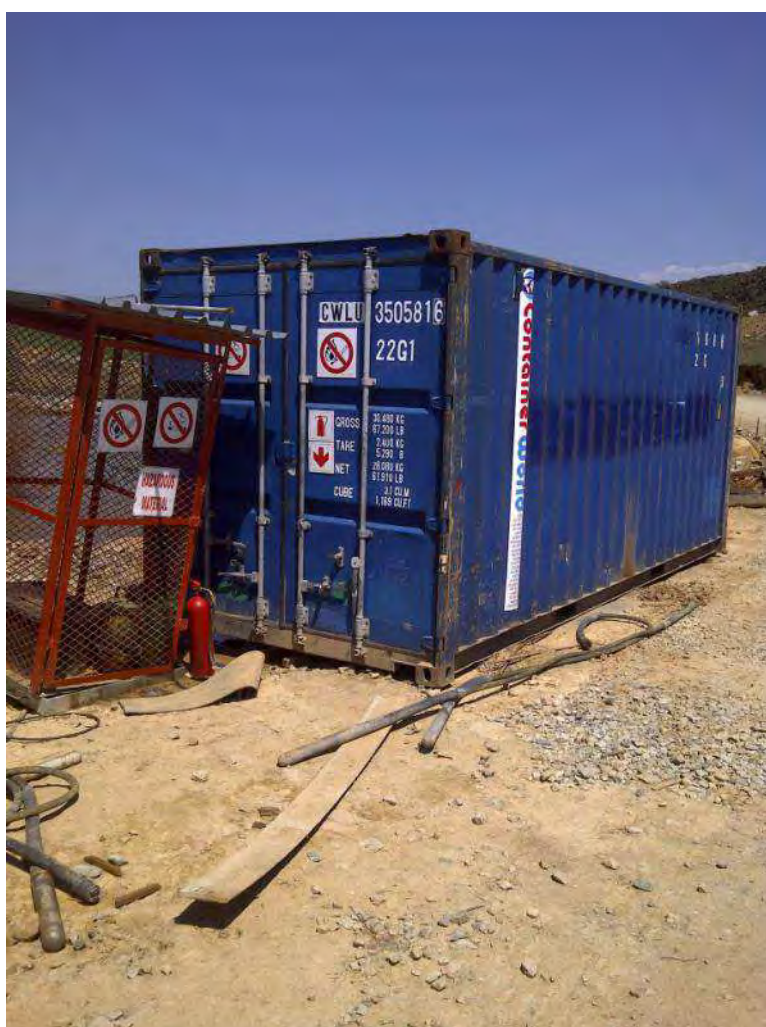
Figure 17: No ventilation of container used for storage of hazardous material
