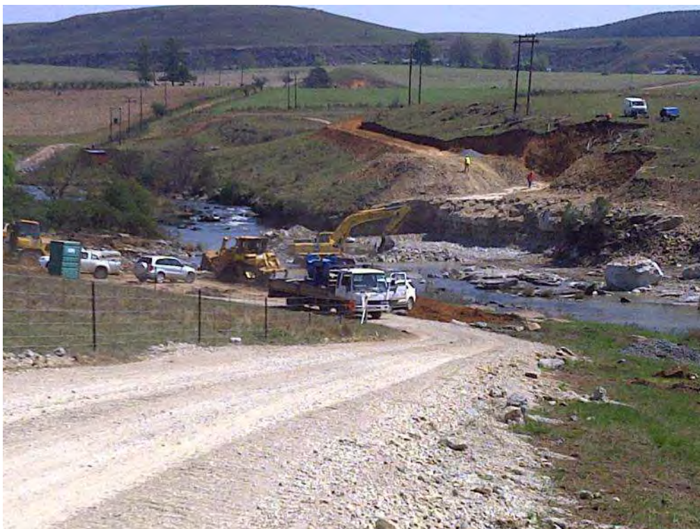
Figure 7: River diversion at fish barrier site
