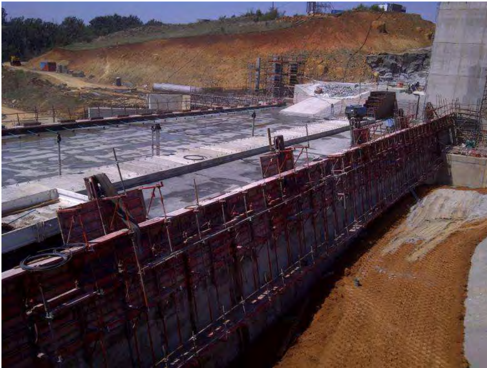
Figure 2: Installation of shutters for the dam base at the dam foundation
