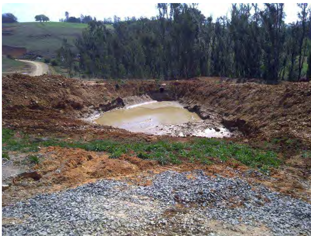
Figure 11: Deepening of sedimentation pond
