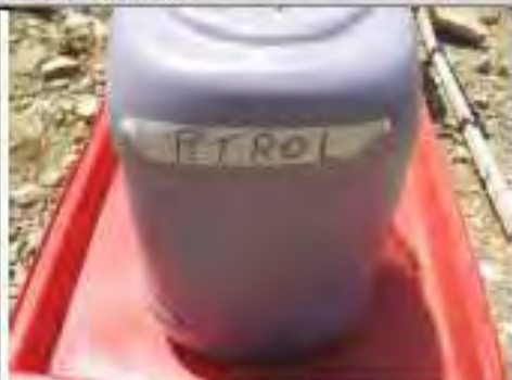
Fig. 2: Use of drip tray under label petrol container at the Right 2 construction site.
