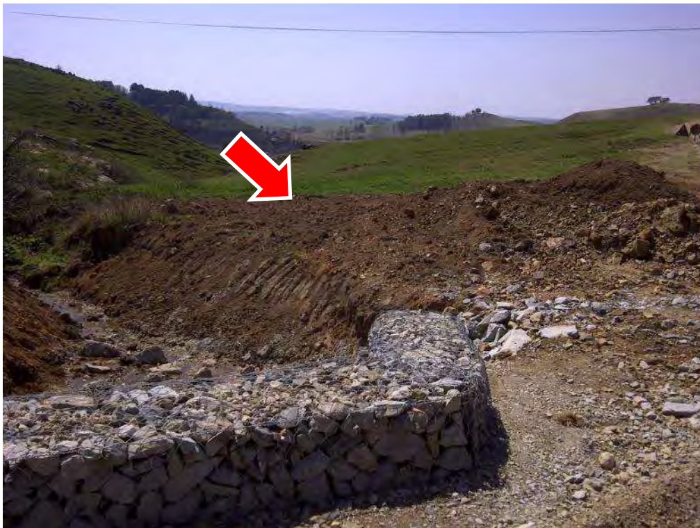
Figure 21: Stockpiling of soil on stream bank
