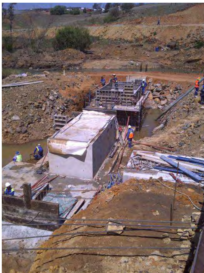
Figure 4: Construction of weir downstream from the dam wall
