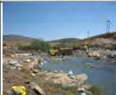
Fig. 3: Equipment crossing the Most River causing sediment to be discharged at the river diversion (fish barrier).
