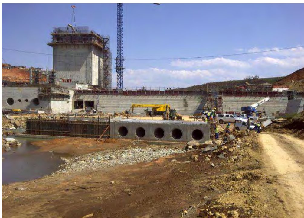
Figure 5: Construction of Route 2 culvert below the dam foundation
