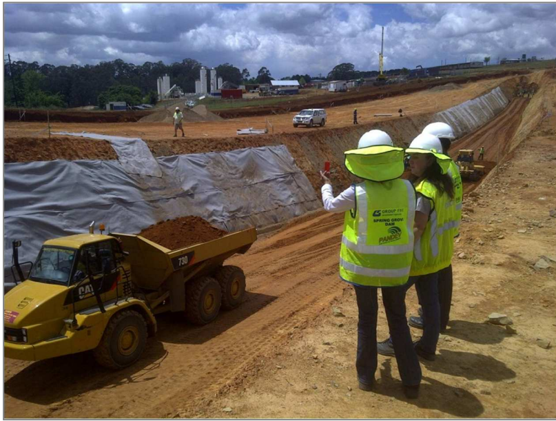
Figure 2: Construction of the earth embankment
