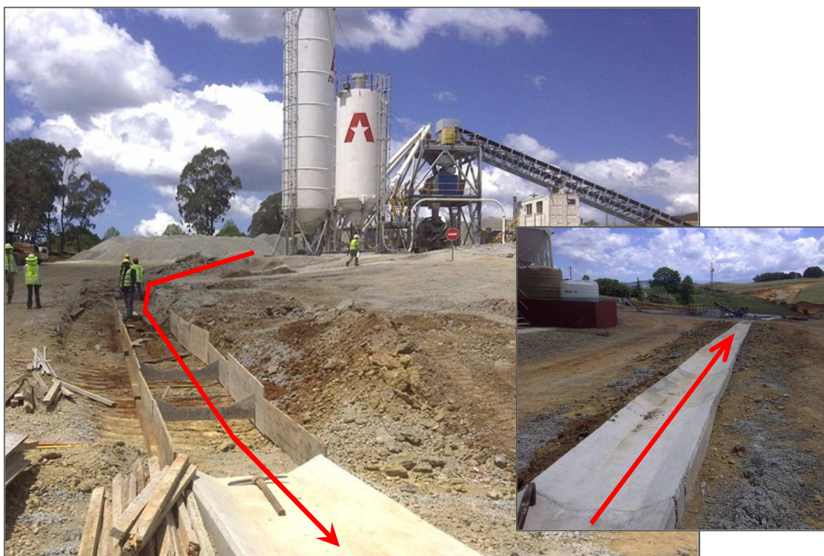
Figure 14: Intervention underway to manage wastewater at batch plant
