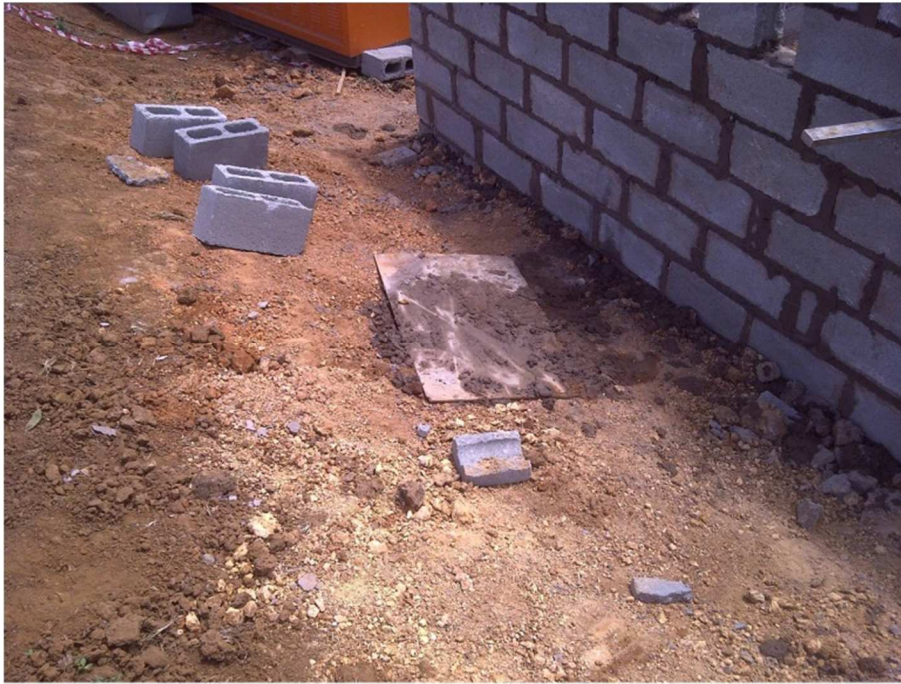
Figure 16: Cement mixing to take place on an impermeable surface
