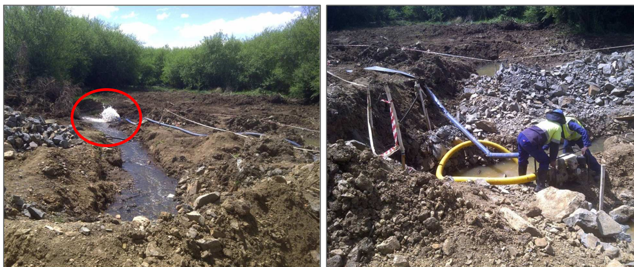
Figure 15: Sedimentation at the watercourse crossing on the D146
