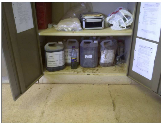
Figure 13: Inadequate storage of hazardous material – area not bunded
