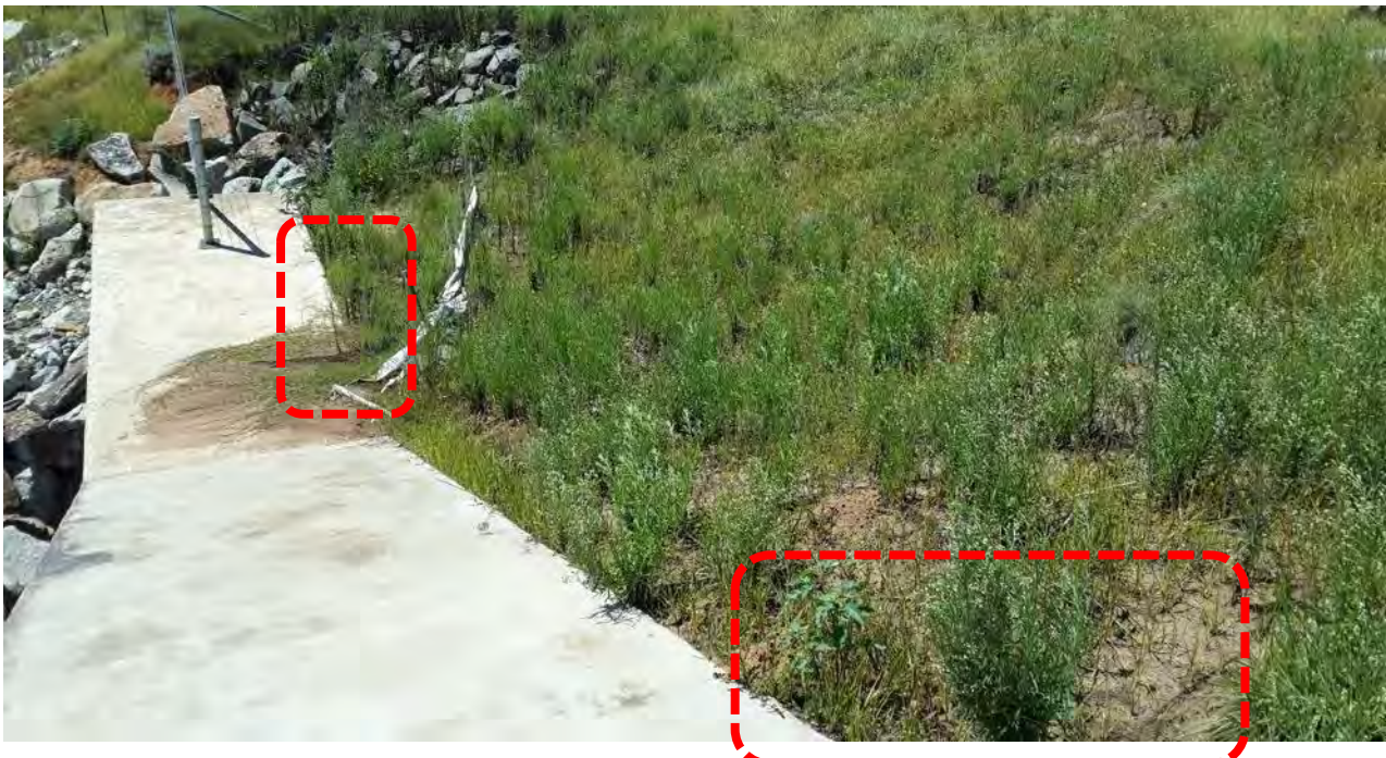
Figure 15: Bare area and cut – fish barrier right bank
