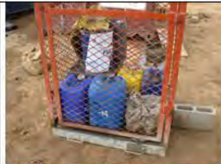
Fig. 18: During this inspection, cage has apparently been relocated to the right bank above the RCC and near the mechanic's container. Although the bunding had been emptied it still is an inadequately sized bund.
