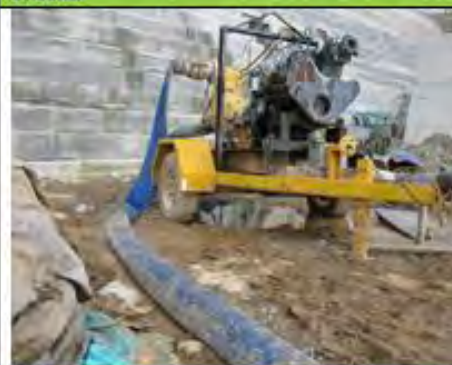
Fig. 22: During this inspection, drip trays were absent from under diesel powered equipment at the river diversion (fish barrier), right bank, and the spillway below dam foundation (above).
