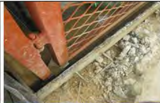
Fig. 17: On 05 December 2012 (date of last weekly inspection), the bunding under the hazardous materials storage cage on the left bank was inadequate in size and close to overflowing with contaminated water.
