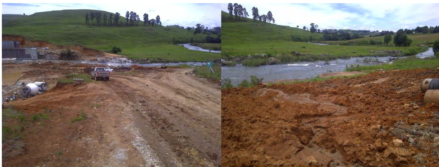
Figure 11: Lack of stormwater management at fish barrier site
