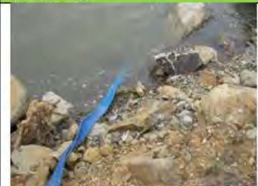
Fig. 19: On 05 December 2012 (date of last weekly inspection), dewatering sock present below the dam foundation at the spillway was not connected to any pump line, rather the dewatering hose pipe was placed directly into the river.
