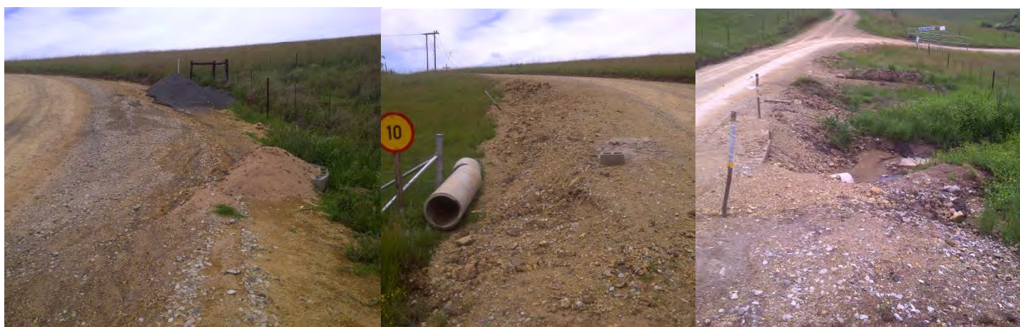
Figure 12: Lack of stormwater management on road approaching fish barrier site
