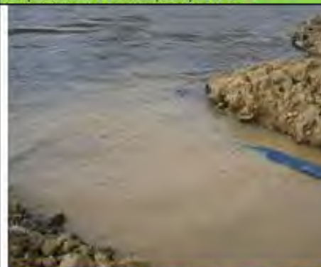
Fig. 20: During this inspection, dewatering sock present below the dam foundation at the spillway was not connected to any pump line, rather the dewatering hose pipe was placed directly into the river and siltation was evident.
